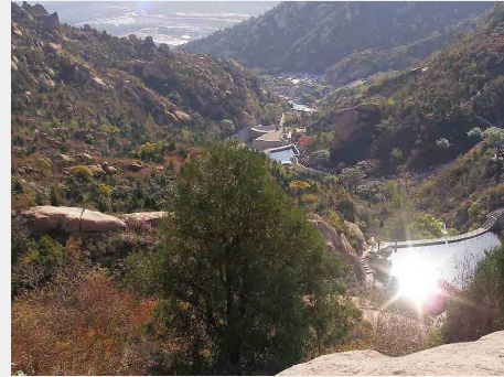
High pressure water delivery
