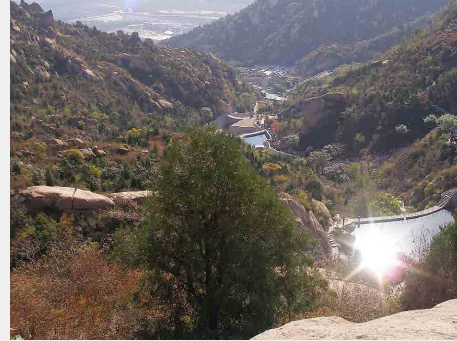
High pressure water delivery
